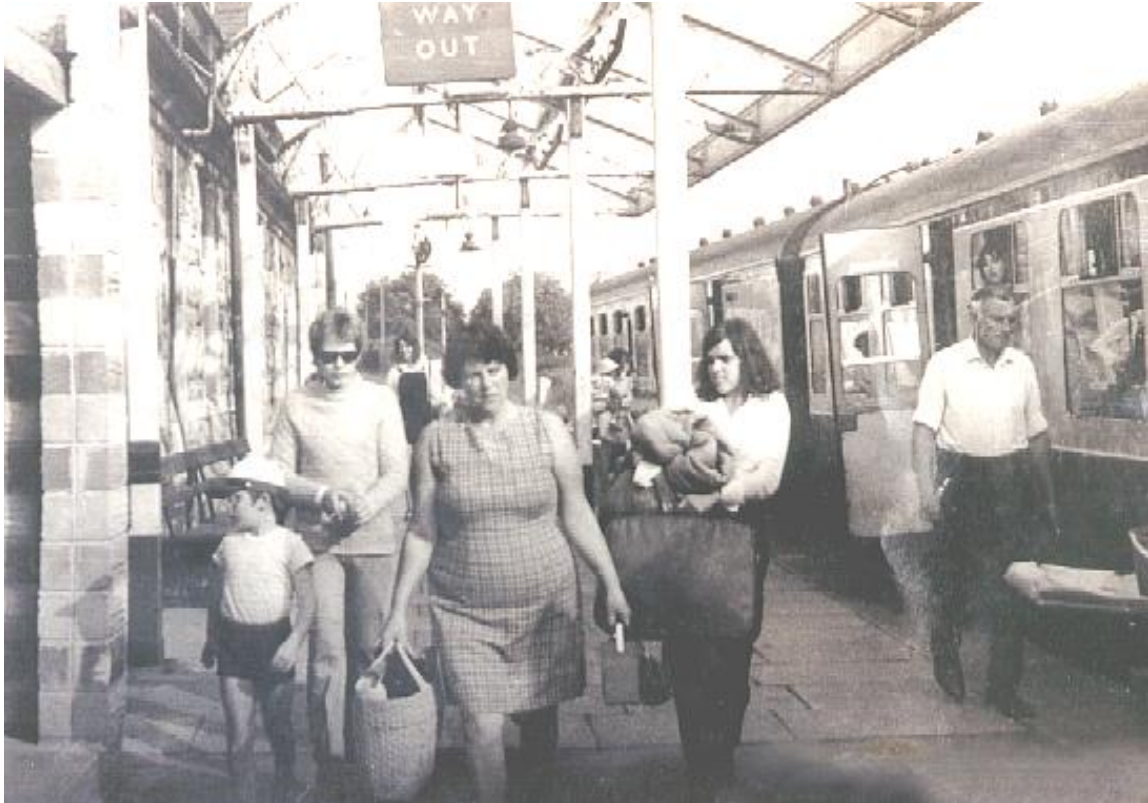
Pembroke Station 1963. Note the wooden pillars supporting the platform canopy and the wall of the 'bus shelter' on the left of the photograph.
